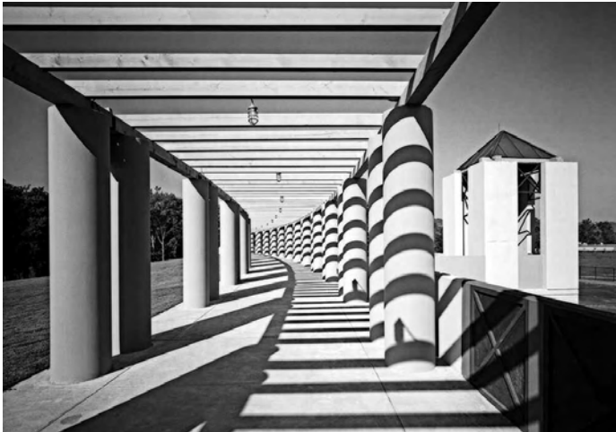
Riverbend Music Center, Cincinnati OH. Designed by Michael Graves. Photographed by Ron Forth ( www.ronforthphoto.com )
